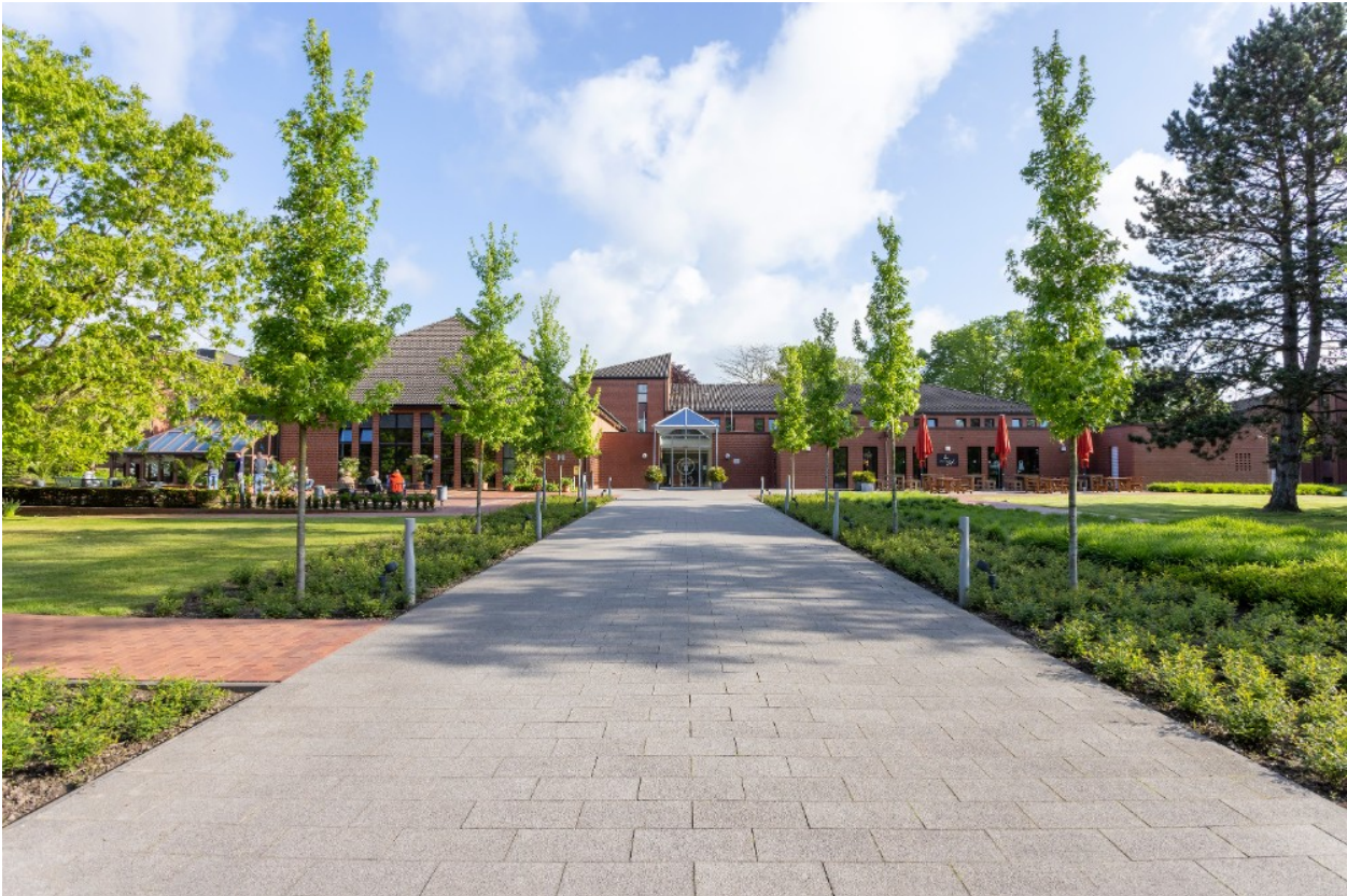
St. Rochus-Hospital Telgte (Haupteingang)
